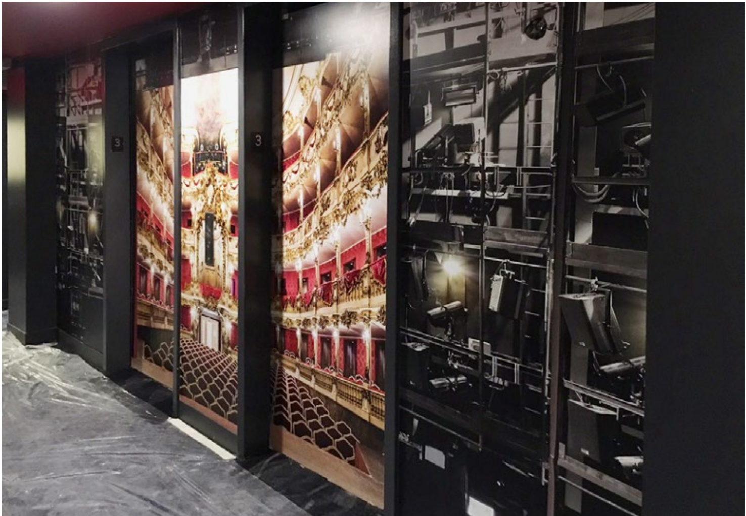
Henri Hotel elevator - Manhattan NY - Work in progress
